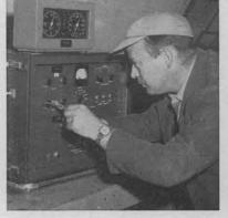
CALIBRATION-W. A. Gustafson, 5226, heads the team of men operating the microbarograph stations surrounding the Nevada Test Site. Prediction of direction and intensity of shock waves is made possible by this program. Chief of the blast studies program is E. F. Cox, 5110.
